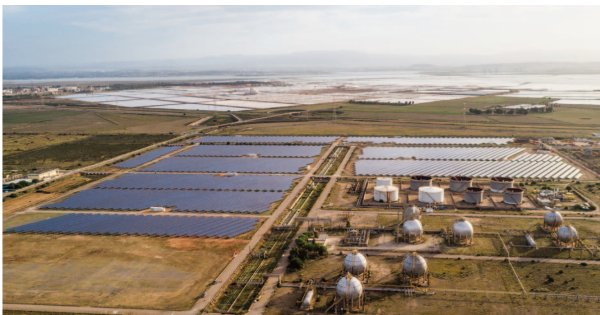
Assemini PV park, 23 MW. Cagliari, Italy.
