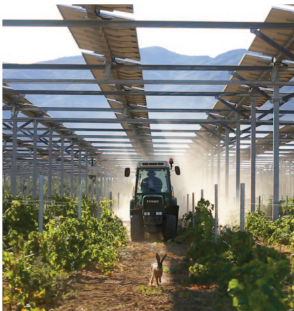
Dynamic shades Agri-PV system, viticulture.
