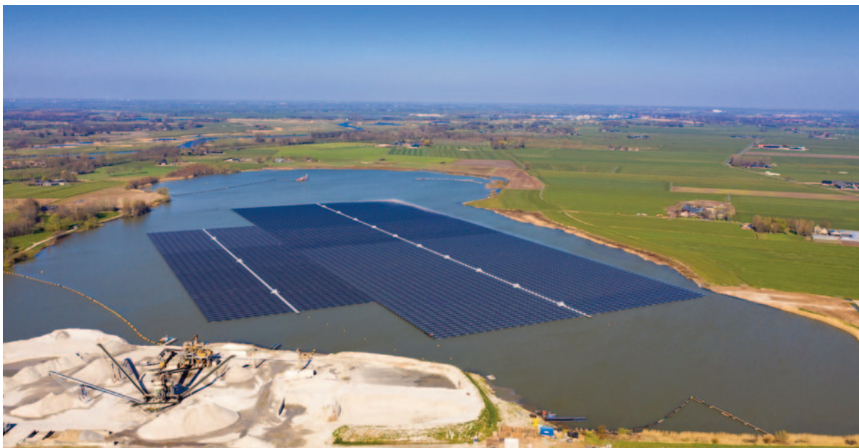
27.4 MW, Bomhofsplas, the Netherlands.
